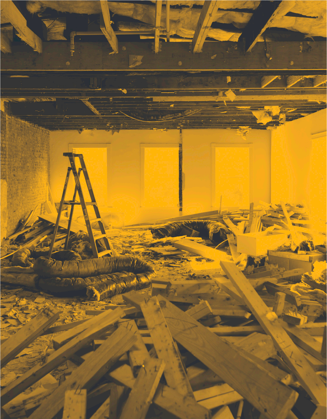
Before: The club level restaurant in the middle of demolition.
